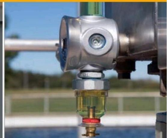
The **Bowl** is a powerful condition monitoring tool, that when coupled with daily inspections can be very effective at identifying, trapping and purging contaminants from your system.
